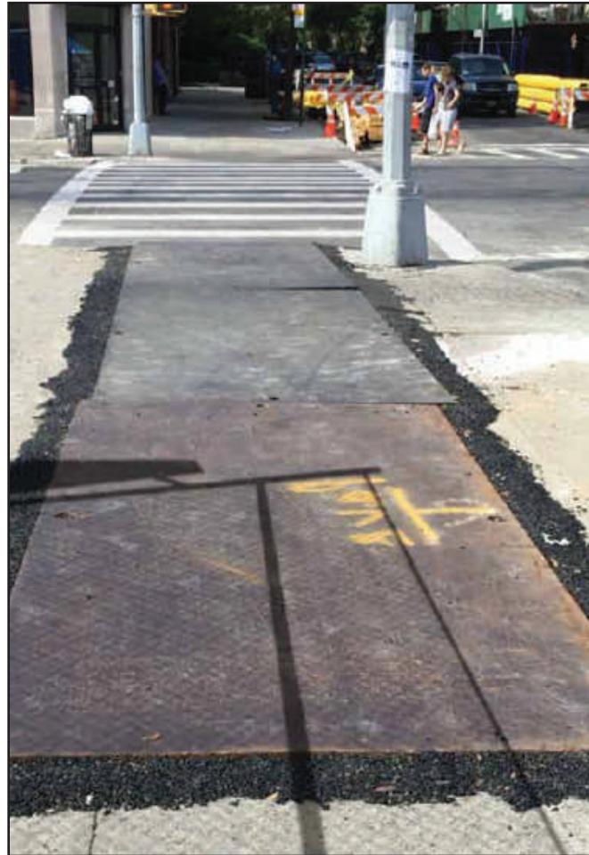
Steel Plates with Cold Patch
